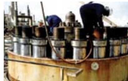
Large methanol reactor with 11" (279,4 mm) studs. Six hours with Superbolt vs. two days with Hydraulic Tensioners.
